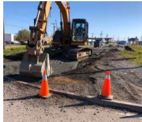
Start of Construction on the Glace Bay Rail to Trail
